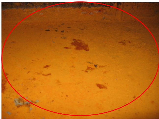
This is the cold air return as seen from the filter change area under the furnace. Heavy corrosion is present and should be addressed by a qualified HVAC technician. The unit should be serviced at regular intervals.
