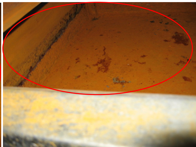
This is the cold air return as seen from the filter change area under the furnace. Heavy corrosion is present and should be addressed by a qualified HVAC technician. The unit should be serviced at regular intervals.
